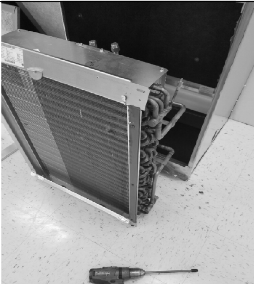
STEP 10. PULL COIL OUT OF UNIT.
