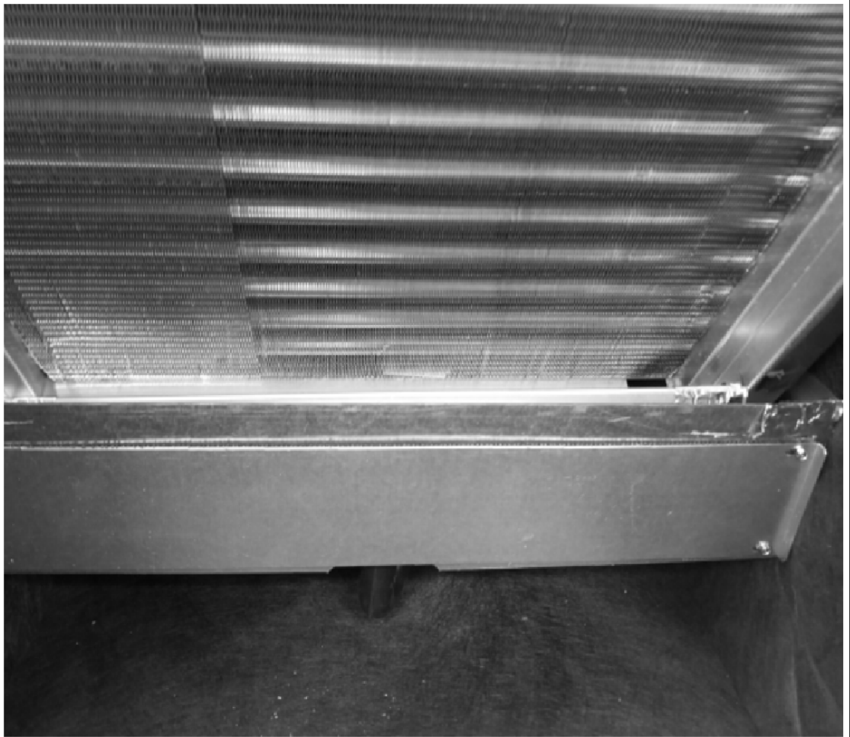
STEP 6. LIFT COIL OFF OF STAND
