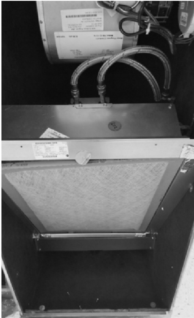
STEP 1. REMOVE BLOWER SHIELD
