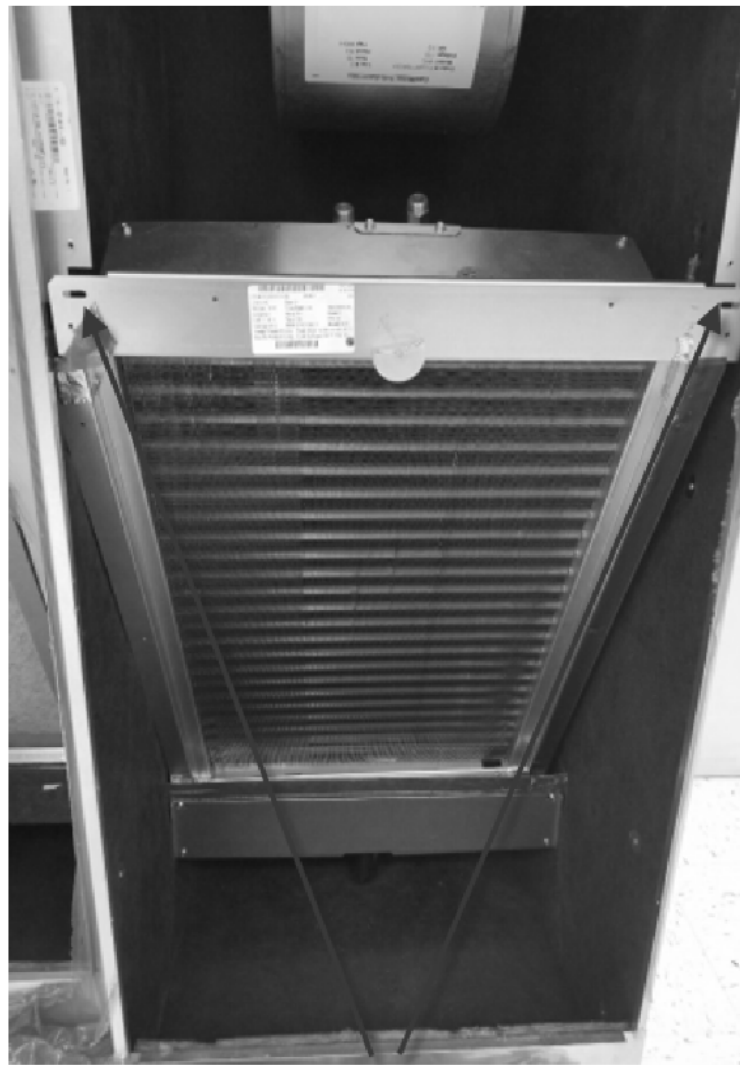
STEP 6. REMOVE 2 SCREWS FROM COIL TOP PANEL TO COIL SUPPORTS
