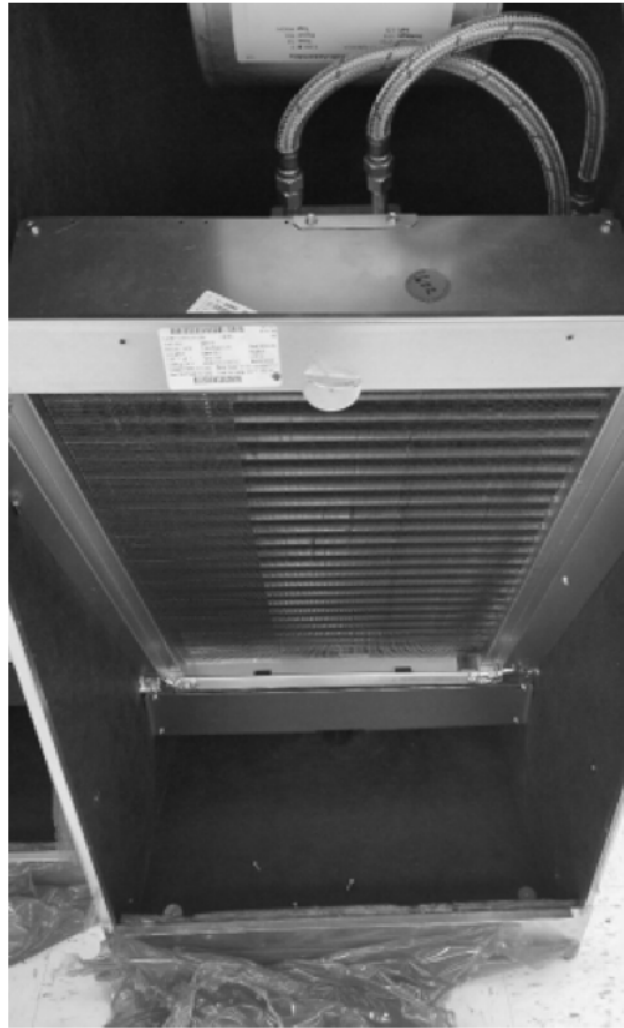
STEP 2. REMOVE FILTER FROM COIL.
