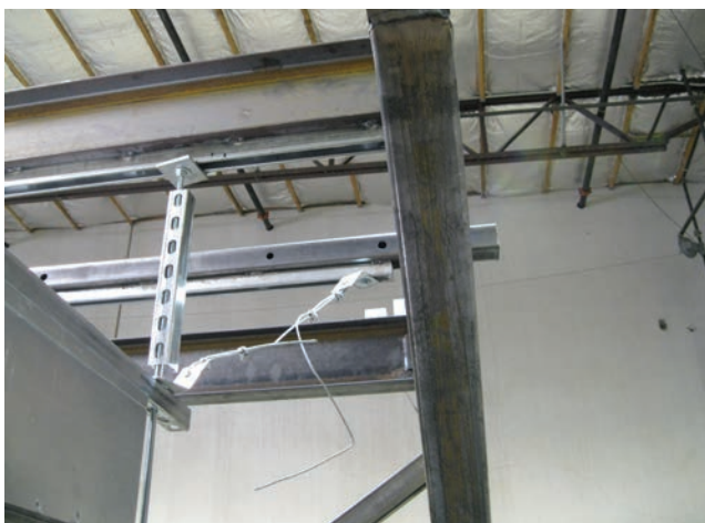
FIGURE 3 – LATERAL SUPPORT COMPONENTS FOR HDD 08-20
