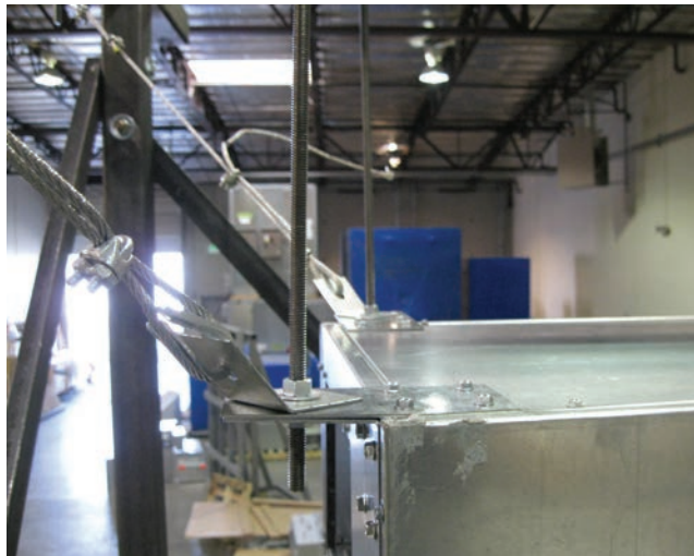
FIGURE 5 – OVERLAPPED FLAT, 90° AND 45° BRACKETS
