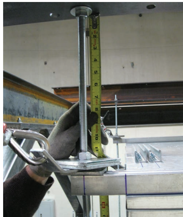
FIGURE 4 – RECOMMENDED LENGTH OF THREADED ROD
