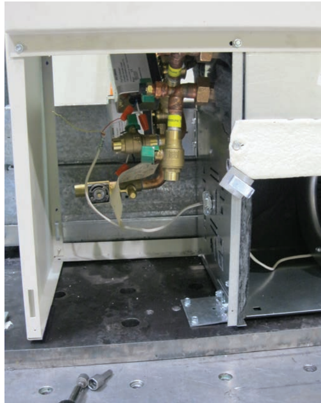
FIGURE 9 – FRONT CLIPS ATTACHED TO UNPAINTED SHEET-METAL FRAME
