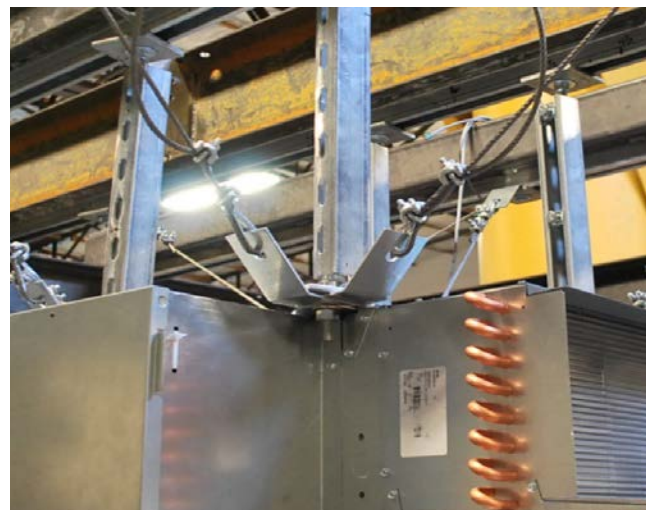
FIGURE 7 – OVERLAPPED FLAT AND 45° BRACKETS
